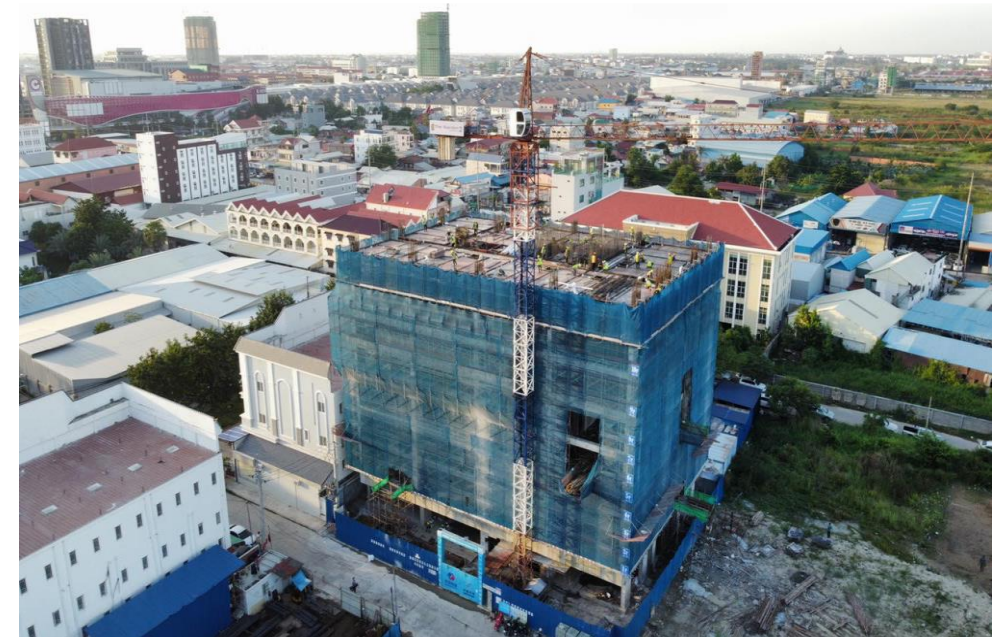
GR2 Construction Progress
